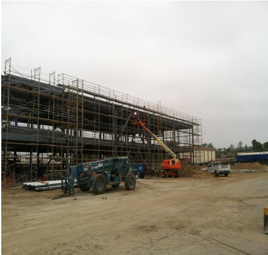
New Building "B" Structural Steel Erection As of 7/1/14
