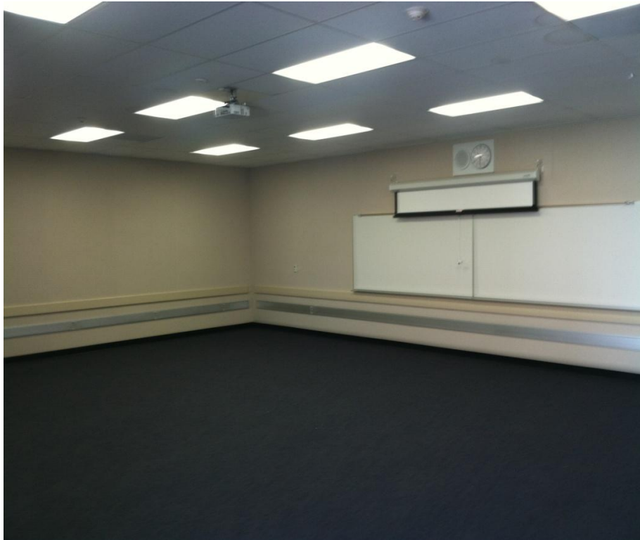
New Classroom Data Raceway, Projector, & Improved Interior Finishes
