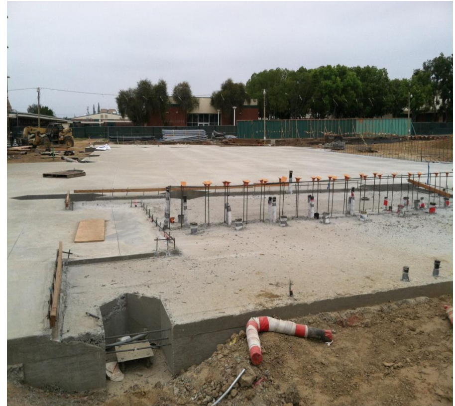
New Building "C" Slab As of 7/1/14
