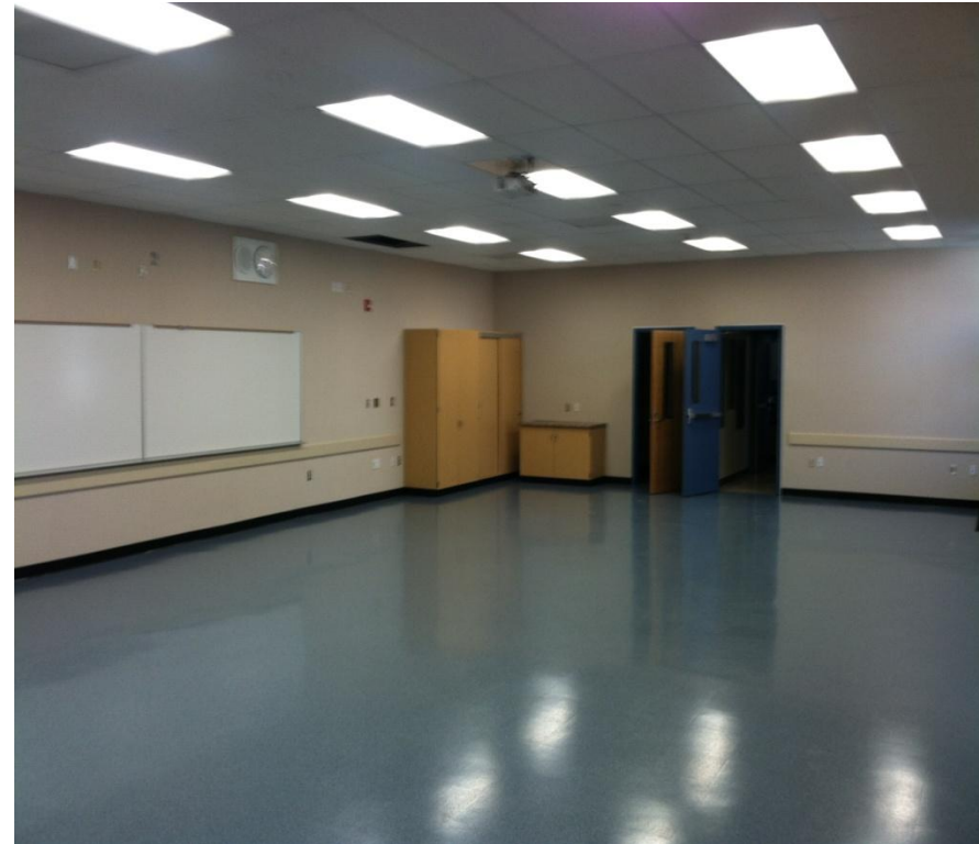
New Classroom Casework, VCT Flooring & Whiteboard
