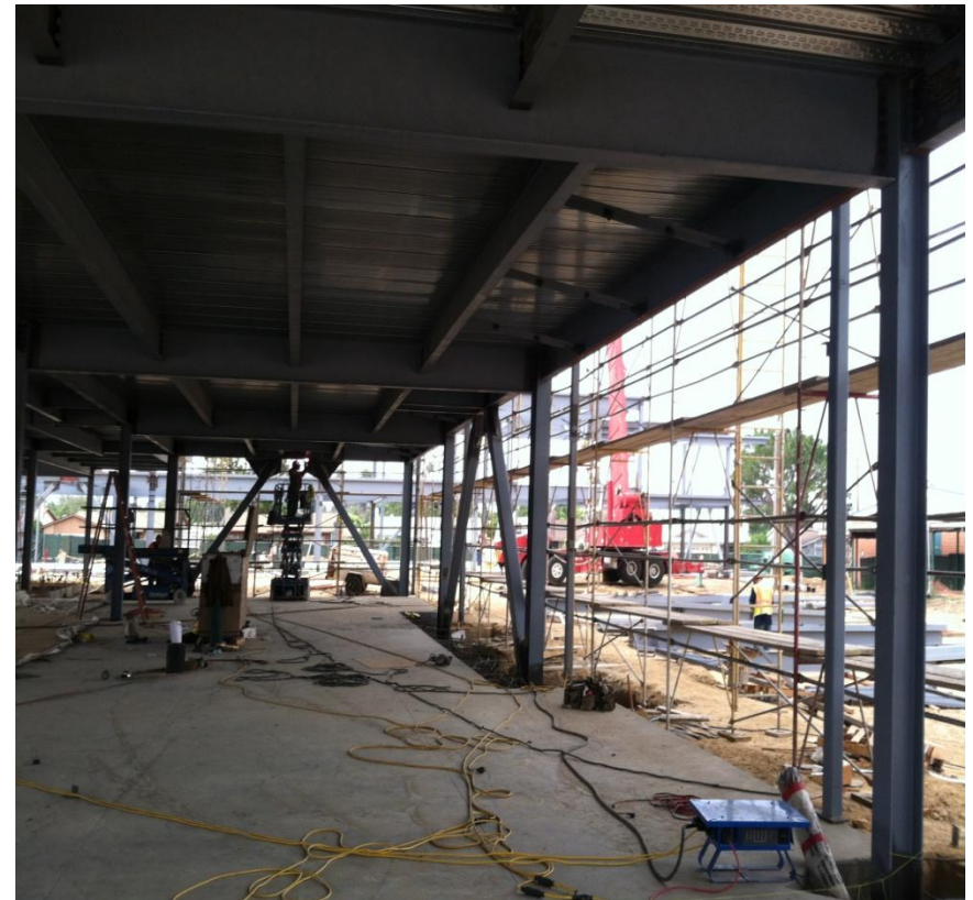
New Building "B" Interior Steel Structure & Decking As of 7/1/14
