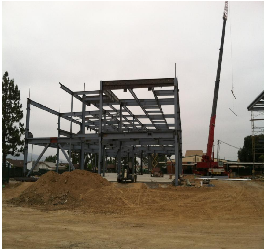
New Building "A" Slab & Steel Erection As of 7/1/14
